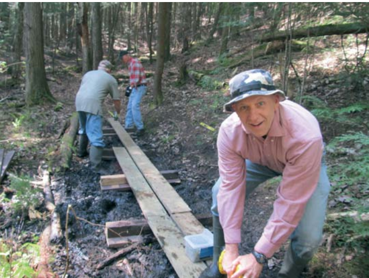
Tim drills deck screws while David and Larry lay out the next section.
